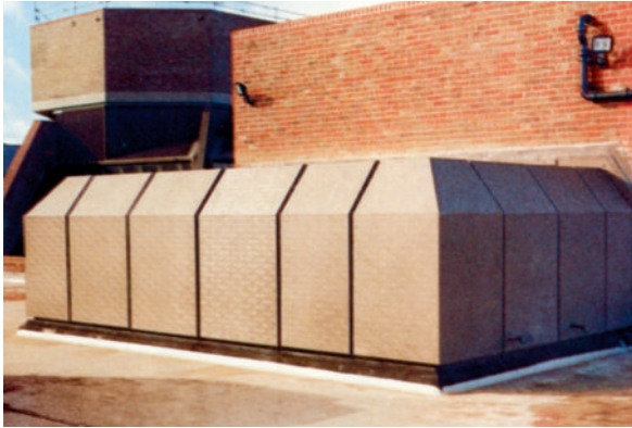
PLANTROOM EXTENSION - Lightweight ALTOS allowed new plant additions to extend onto low load bearing roof and sealed to existing brickwork
