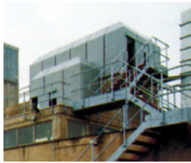
A split level ALTOS housing with double doors for plant access and 'lift-off' roof serving a nuclear power station
