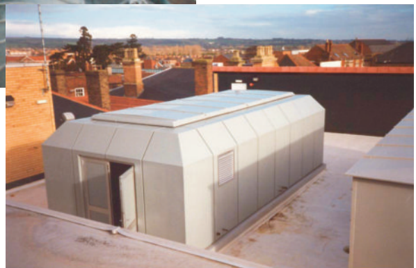
Rooftop ALTOS modular housing
