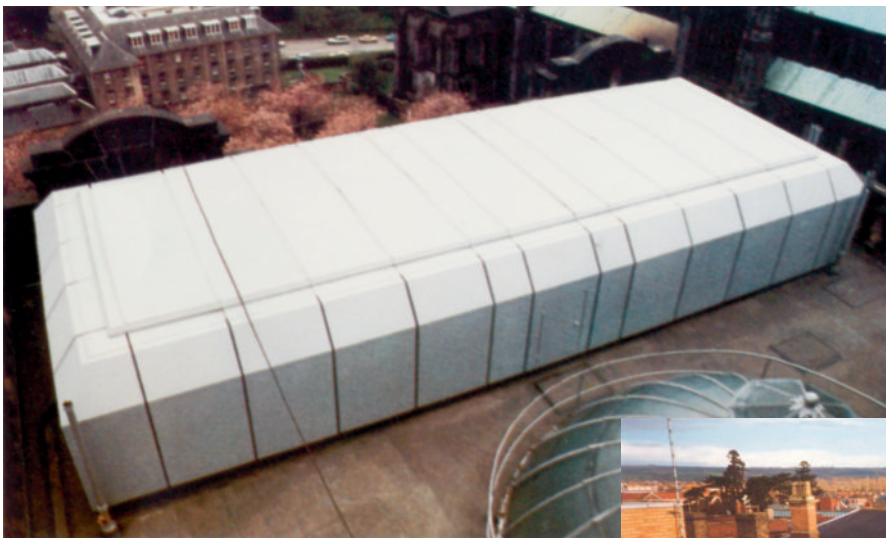
Extensive new low-profile PLANT ROOM on old building to accommodate up-dated services
