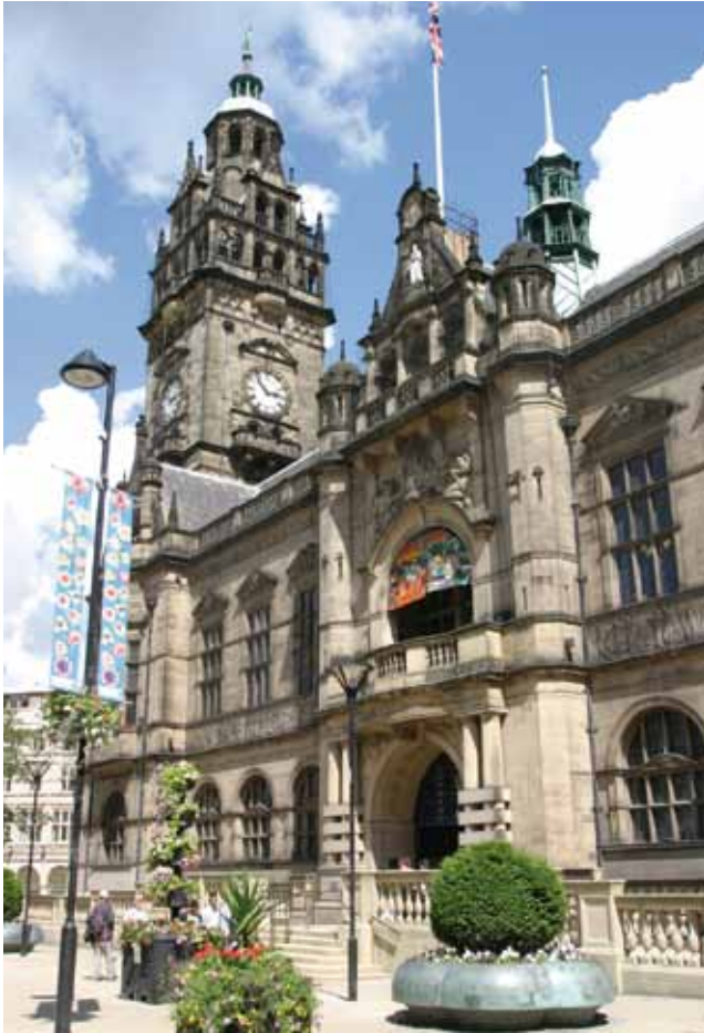
The search for a tower block, for use as premises for the Sprinkler Coordination Group's retrofit project, took the SCG to Sheffield Town Hall, for discussions with the City Council. It was agreed among the parties that a candidate tower block could be found among those at Callow Mount, being City Council properties managed by Sheffield Homes. (Photo by permission of Sheffield City Council.)
