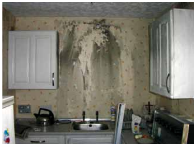
A fire in the kitchen of a sprinklered flat in South Ayrshire was extinguished by a sprinkler.
